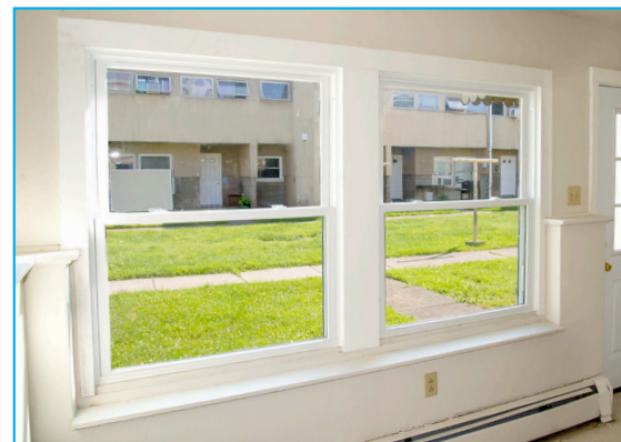
Pictured above, new windows installed at SHA's Riverside Apartments that feature modern trim board frames which replace wood frames without the need for painting. At right, work crews are on-site at Jackson Terrace Apartments installing new doors.
